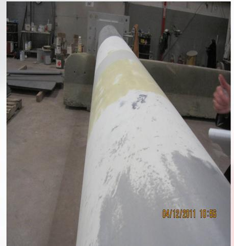
Filling Work Over Galvanized AESS Steel On A Light Pole
